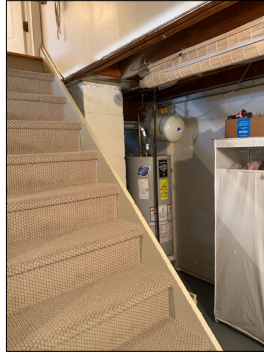
Missing safety/handrail
