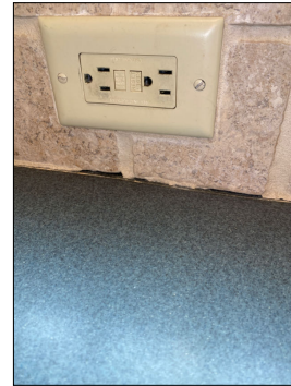
Caulking failure
