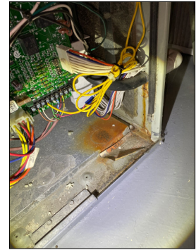
Localized corrosion
