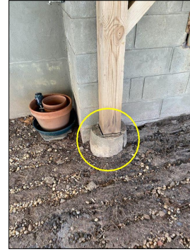
Cracked footing
