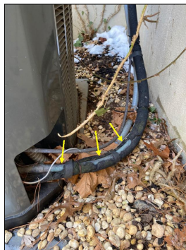
Damaged/missing insulation
