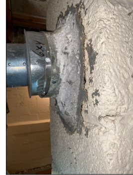
Junction deterioration
