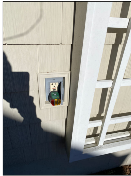
Incorrectly wired
