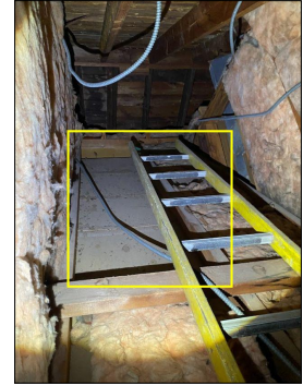
Missing insulation
