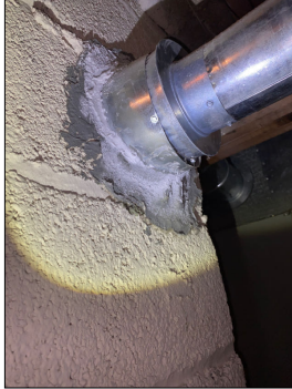
Junction deterioration
