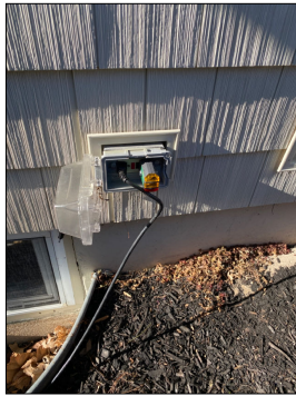
Incorrectly wired
