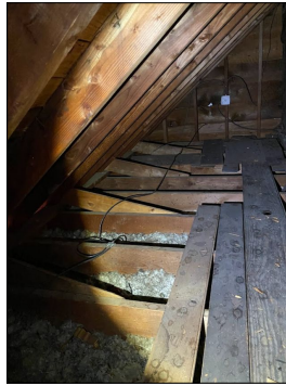
Insufficient insulation
