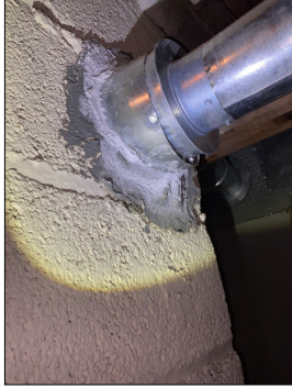
Junction deterioration
