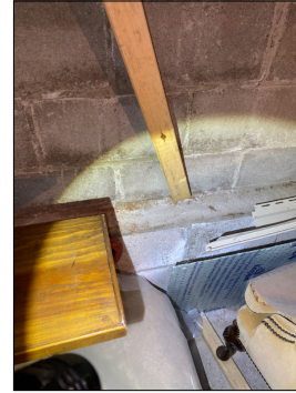
Water staining / efflorescence
