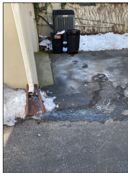
Discharge too close to foundation
