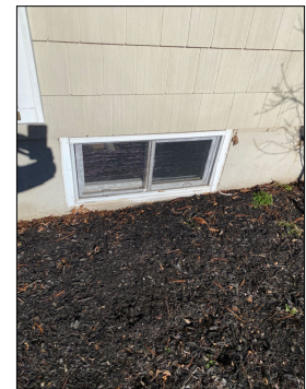
Poor foundation clearance
