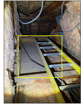
Missing insulation
