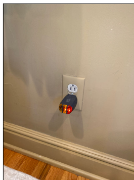
Incorrectly wired receptacle, #2
