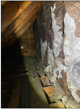
Incorrectly installed insulation
