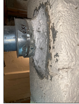
Junction deterioration
